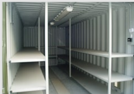
Fitted shelving and electrics
