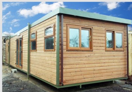
Thermowood timber external cladding
