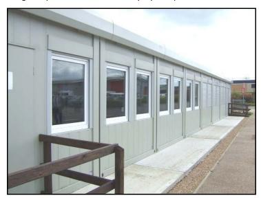
These office cabins can be used either as individual units or in combinations for modular buildings. By leaving out wall panels and installing partition walls any room sizes can be created.
